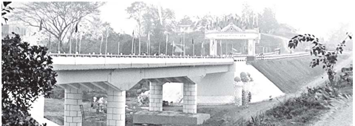
Pyinyaung Bridge on Meiktila-Taunggyi-Kengtung-Tachilek Road.—MNA
