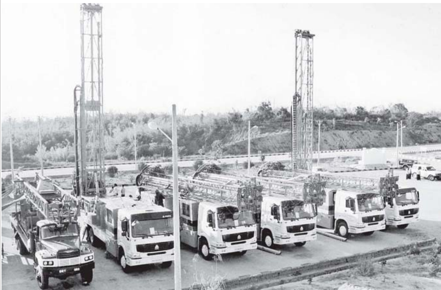
Arrival of RG truck-mounted drilling rigs manufactured by the People's Republic of China at worksite.
