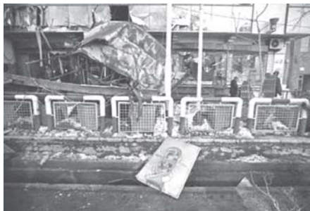
A view of the damaged entrance of the City Centre shopping mall after a suicide bomb attack, in Kabul on 14 Feb, 2011.—INTERNET
