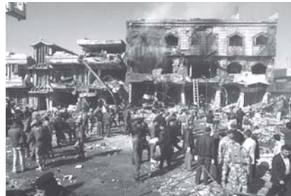
Security forces, emergency responders and civilians stand near a destroyed building after a car bomb attack in Kirkuk, 290 kilometres (180 miles) north of Baghdad, Iraq, on 9 Feb, 2011.
