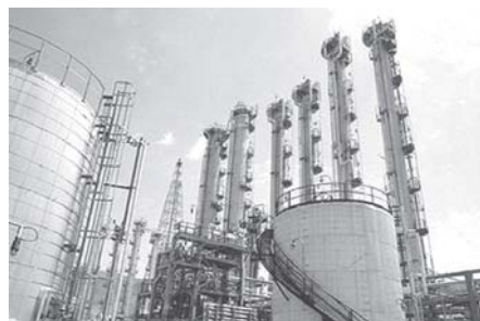
A general view of a heavy water plant in Arak, 320 kms south of Teheran in 2006. Iran's atomic body claimed on Thursday it has mastered the technology of nuclear fusion, in a declaration on the eve of the 32 nd anniversary of the revolution.—INTERNET
