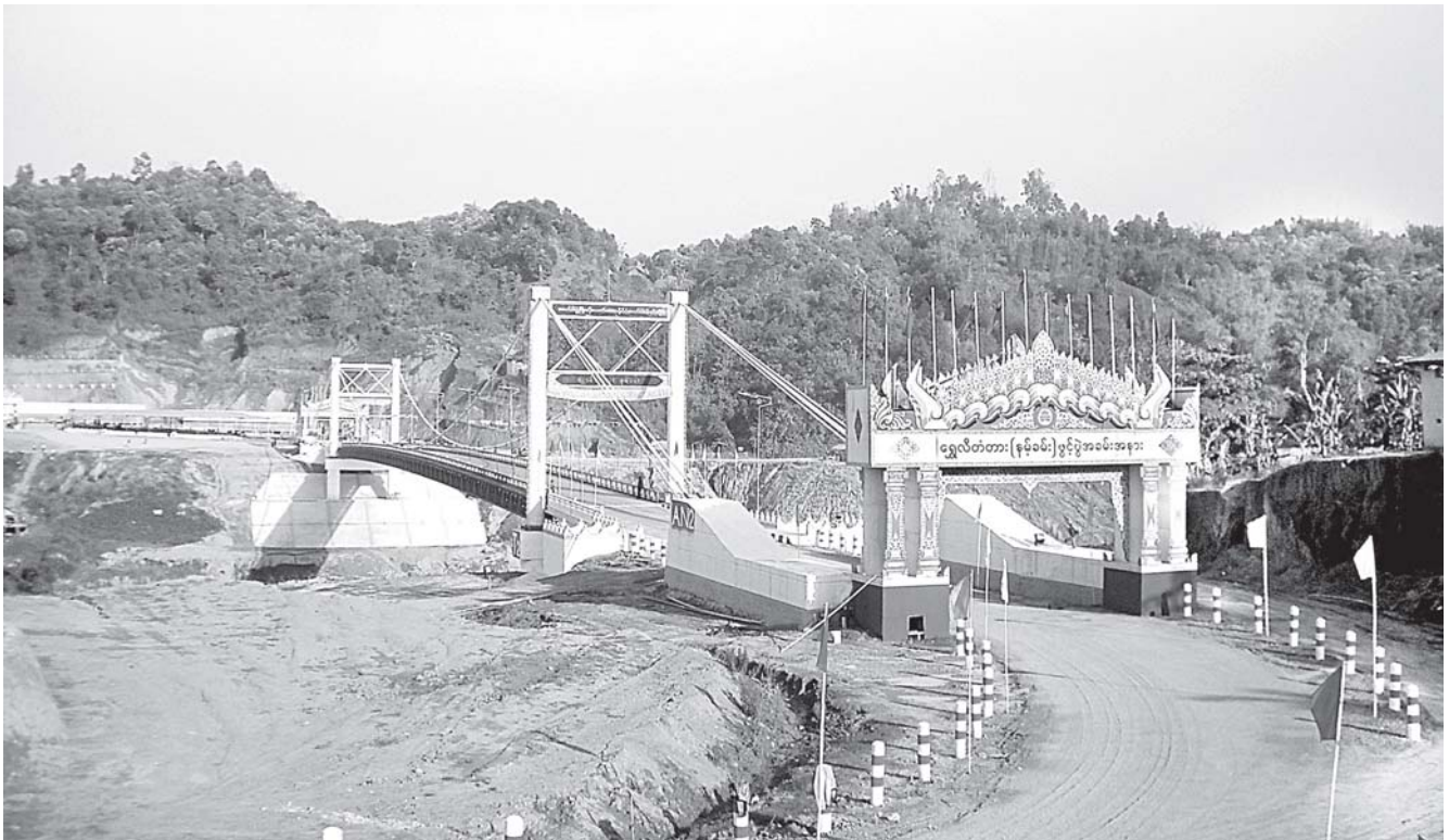
Photo shows Shweli Bridge (Namkham).
