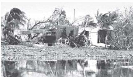
A beachfront home lies in ruins, on 5 February, after Cyclone Yasi devastated the coastal hamlet of Hull Heads.—INTERNET
