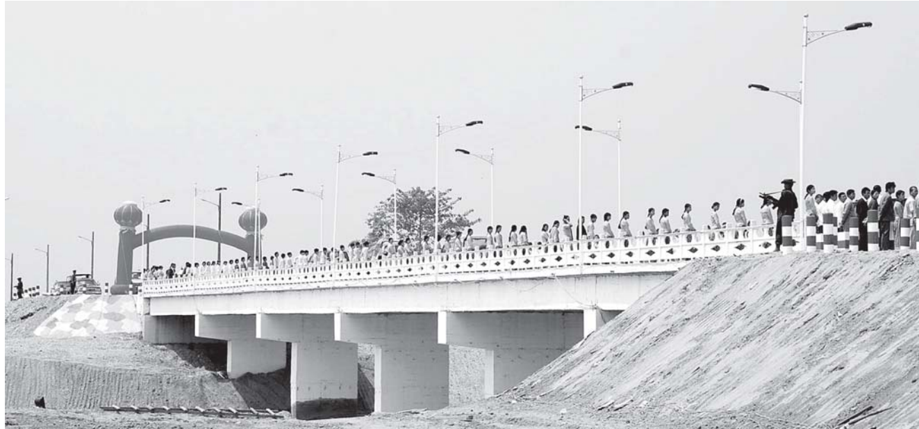
Warazup Bridge No. 2 on Myitkyina-Nanti-Tanai Road.
