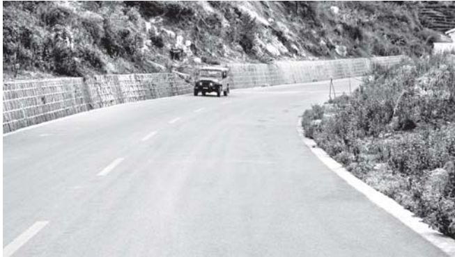
Photo shows part of Myitkyina-Waingmaw-Hsadon-Kanpaikti Road that contributes to smooth and swift flow of passengers and commodities in Kachin State.
