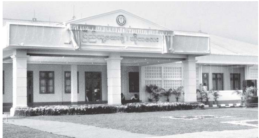
New People's Hospital (100-bed) in Bogale Township.
