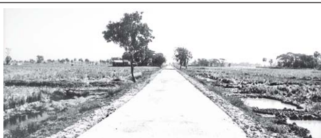
Newly-built Nibban Road is designed for smooth transport in Dala Township.
