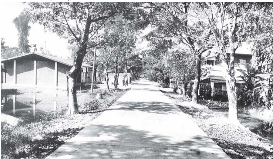
The 7000 feet long Sinbyushin concrete road linking Bayintnaung, Tabinshwehti and Kyansittha wards in Dala Township.
