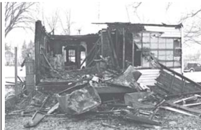
The burned home of Lamar D Moore is shown at 14294 Sorrento Street in Detroit on 25 Jan, 2011. Detroit Fire Capt Kwaku Atara says the fire was called in at 3:14 am Tuesday, and its cause is undetermined. Moore opened fire inside the Detroit Police Department 6th precinct on Sunday, wounding four officers including a commander before police shot and killed him.
