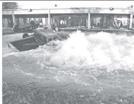
A water main break is seen at an industrial park next to the Capital Beltway in Capitol Heights, Md, on 24 Jan, 2011. The break outside Washington has sent water pouring from a 54-inch pipe, prompting the closure of the inner loop of the Capital Beltway in Maryland and snarling morning traffic.—INTERNET
