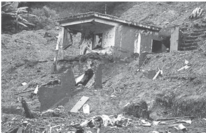
A destroyed house at Campo Grande neighbourhood in Teresopolis, some 100 km from Rio de Janeiro. The Brazilian military sent troops and helicopters Sunday to rescue stranded survivors of floods and landslides that killed more than 625 people but the operation was stymied by more bad weather.—INTERNET
