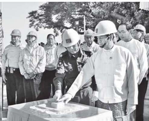
Commander Brig-Gen Ye Aung and Minister U Khin Maung Myint lift first truss of Ayeyawady Bridge (Pakokku). MNA
