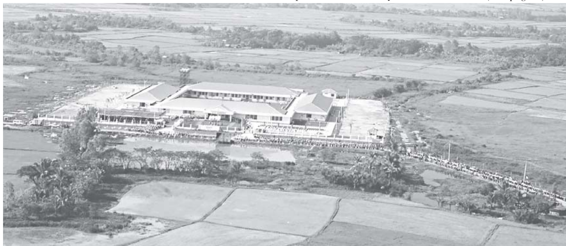
Aerial view of 100-bed Bogale Township People's Hospital.—MNA
