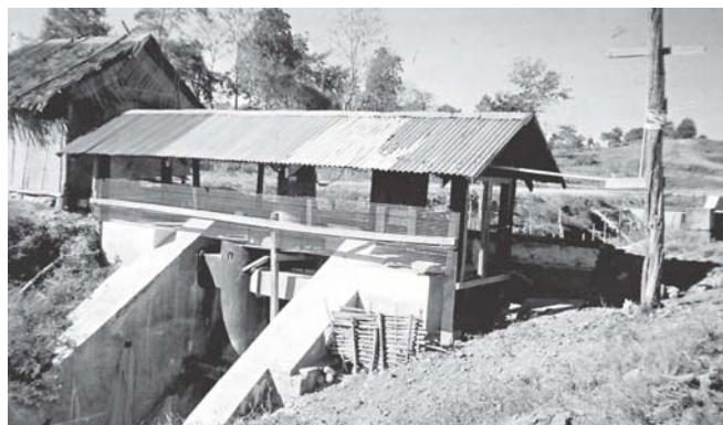
A small-scale hydropower plant in the main canal of Maday Dam.
