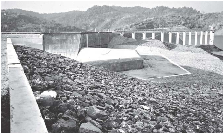
Maday Dam seen with the background of mountain ranges.
