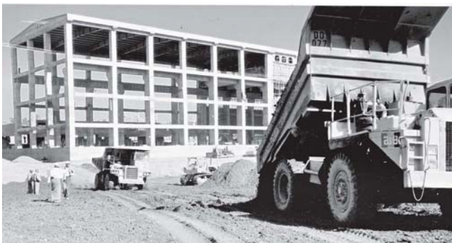
Power house and earth work being carried out with heavy machinery.
