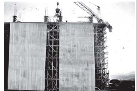
Construction of intake structure seen at Kyee-Ohn Kyee-Wa Multi-Purpose Dam Project.
