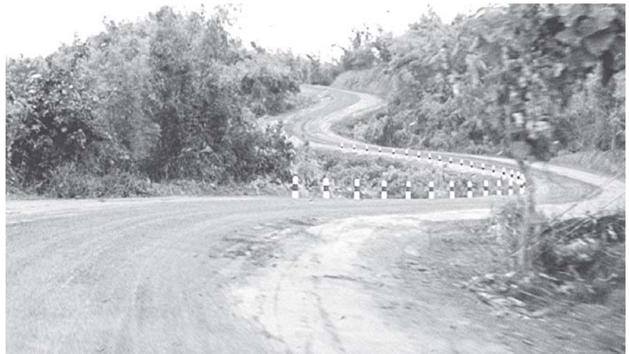
Photo shows a road section of Taikkyi-Phaunggyi-Bago Road.
