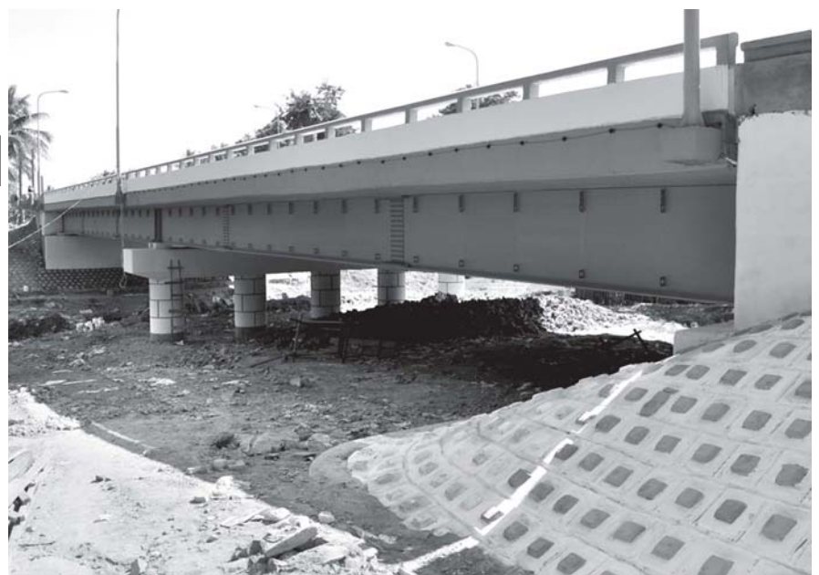
Kyweshin Bridge Project (180 feet long) is nearing completion.
