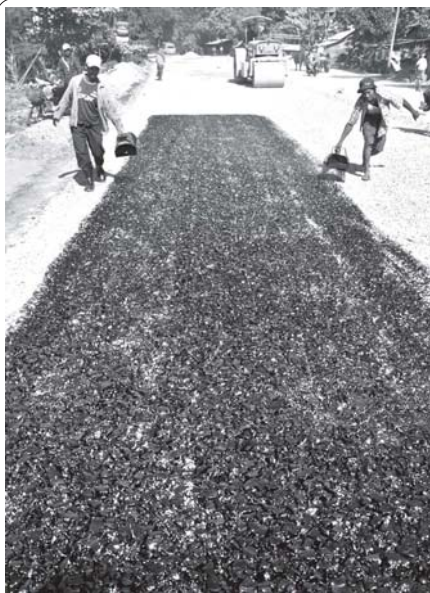
A section of Pyinmana-Taungnyo Road is being tarred.
