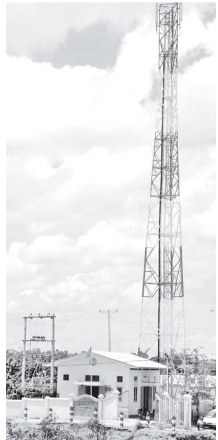
GSM radio station and its tower seen in Chauk Township.
