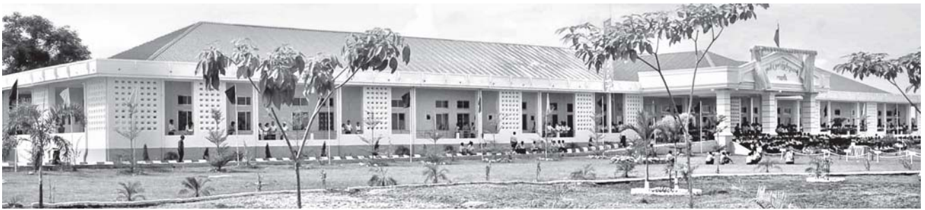
The 200-bed general hospital seen in 3rd-Mile satellite area of Labutta Township.
