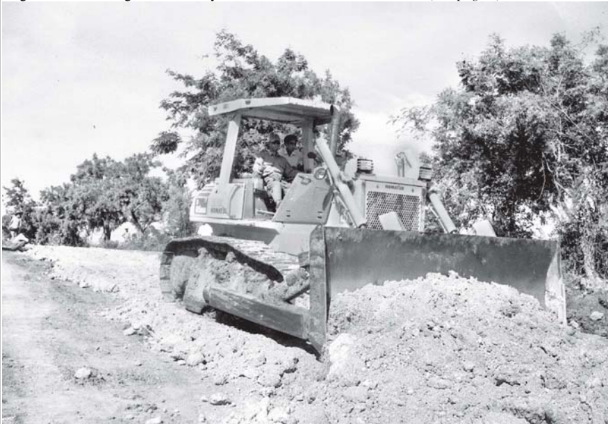
A bulldozer is at work for maintenance of Kanbalu-Taukkashat Road.
