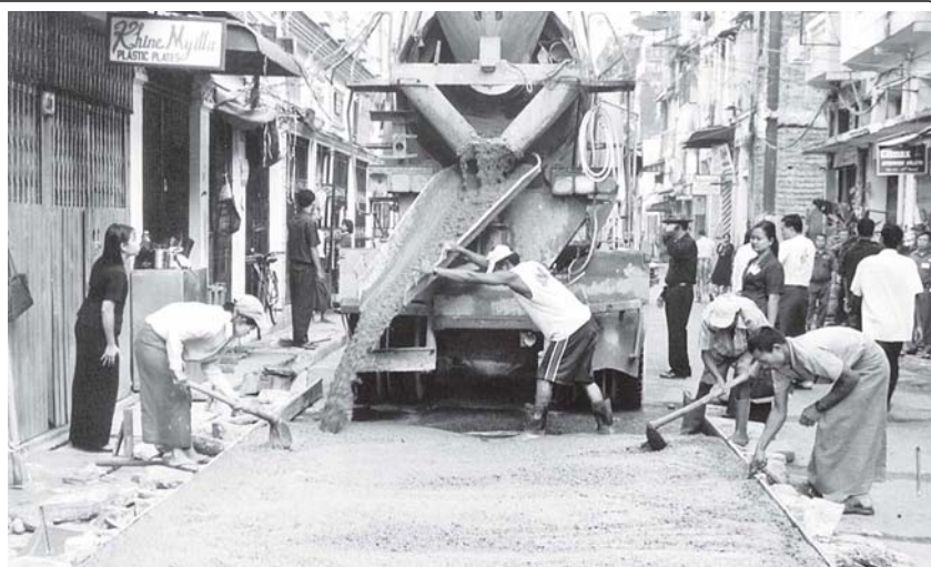
Photo shows workers paving a concrete road in Yangon municipal area.
