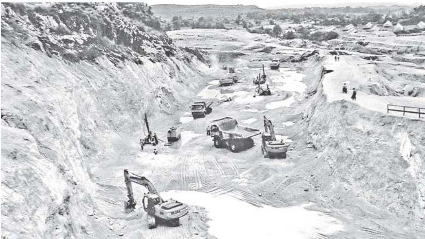
Pwekauk Diversion Weir under construction with the use of heavy machinery.
