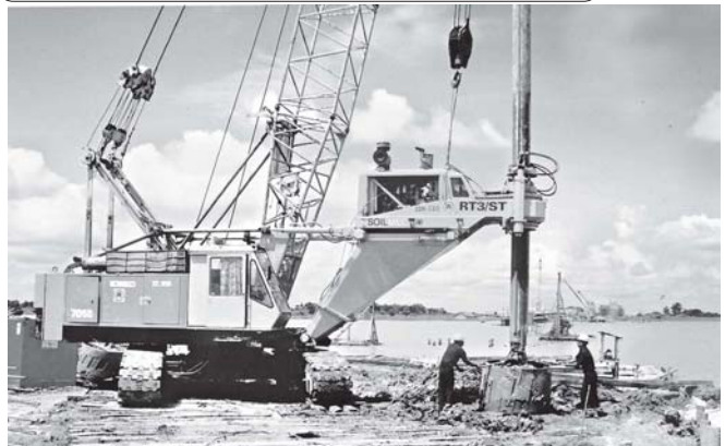
Photo shows digging of bored pile at RP-1 of Ayeyawady Bridge (Nyaungdon) with the use of heavy machinery.
