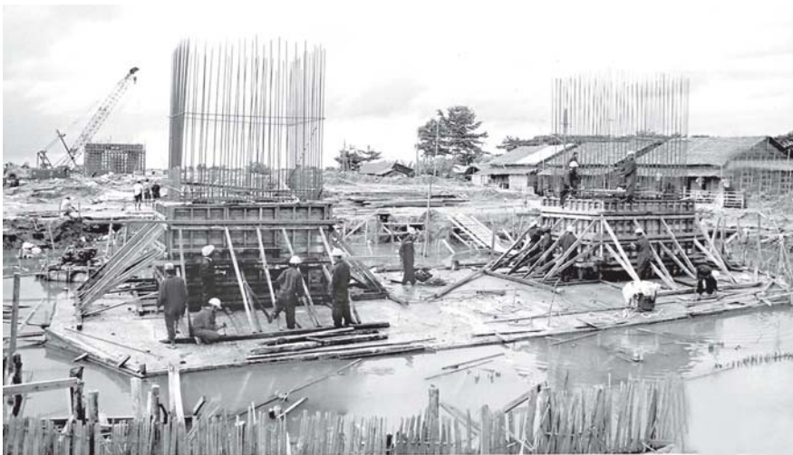
Shaft works at RP-8 of Ayeyawady Bridge (Nyaungdon).
