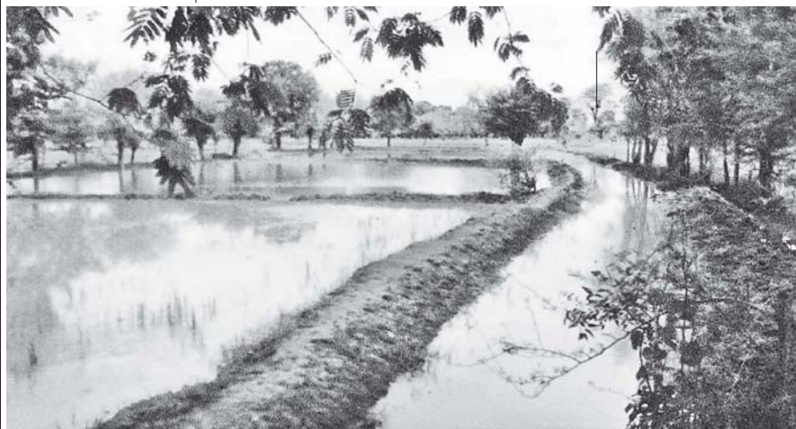
Irrigation water is supplied to paddy fields through the secondary canal.
