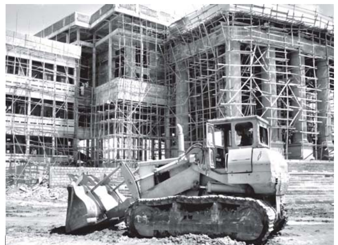
A bulldozer in action making the ground even in the project site.
