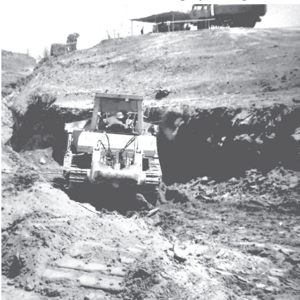
Heavy machinery is in use to build spillway of Mokkha Dam.
