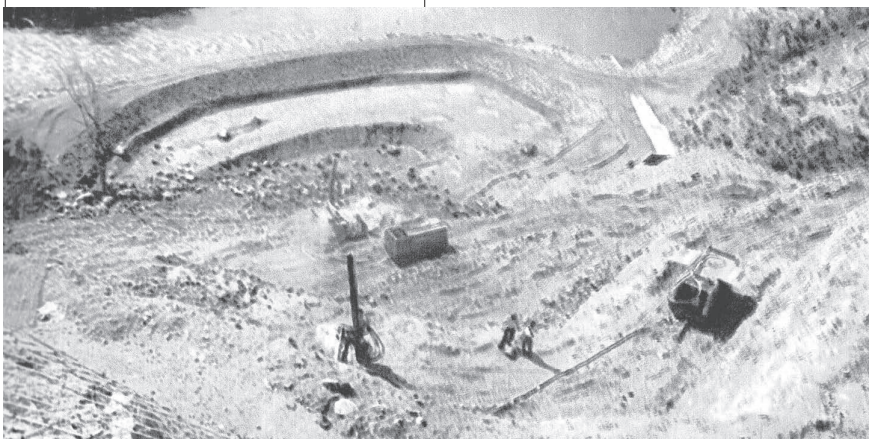
Approach water intake tunnel No (4) of Belu Creek No. 3 Hydropower Project under implementation.
