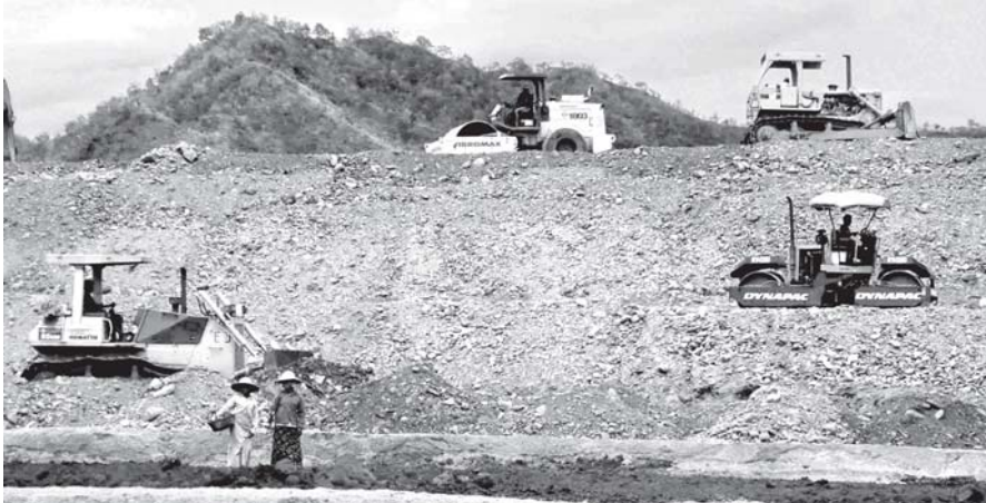
The main embankment of Myogyi multi-purpose dam under construction.
