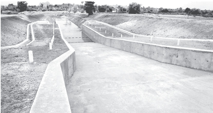
Photo shows progress in construction of RC type spillway.
