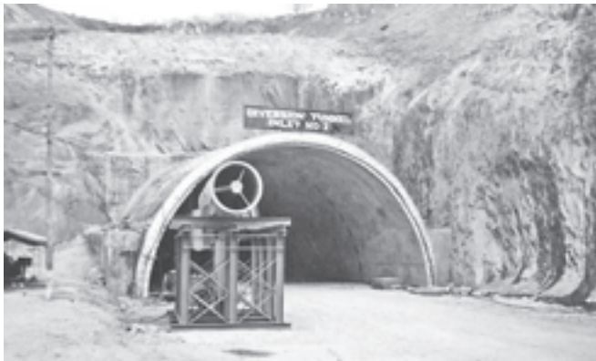
Constuction of diversion tunnel inlet No. 2 of Manipura multi-purpose dam.
