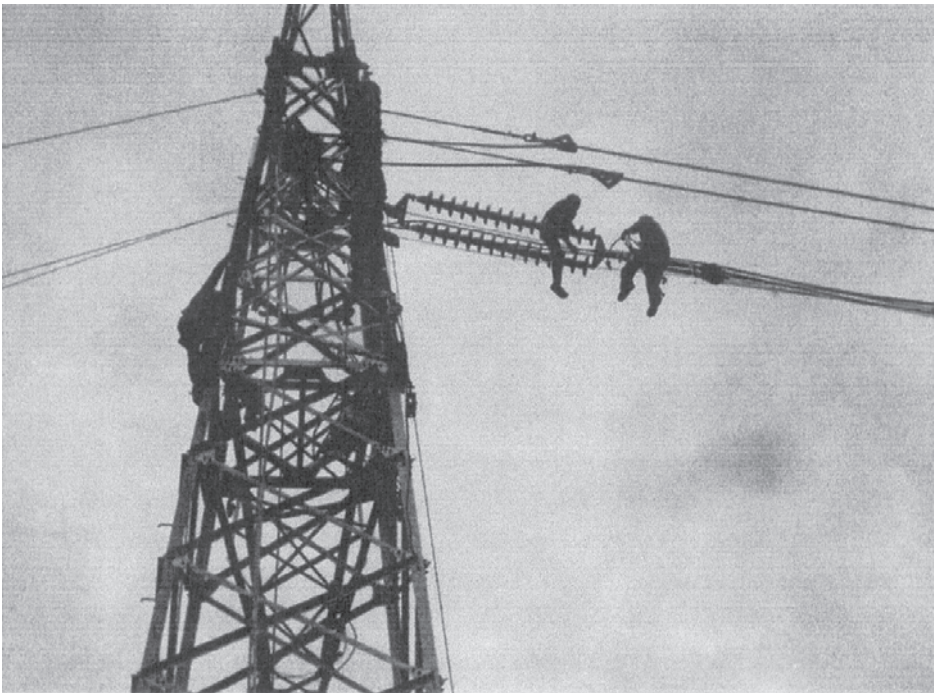
Power line installation of 230 KV at Upper Paunglaung-Nanhkio power grid in progress.
