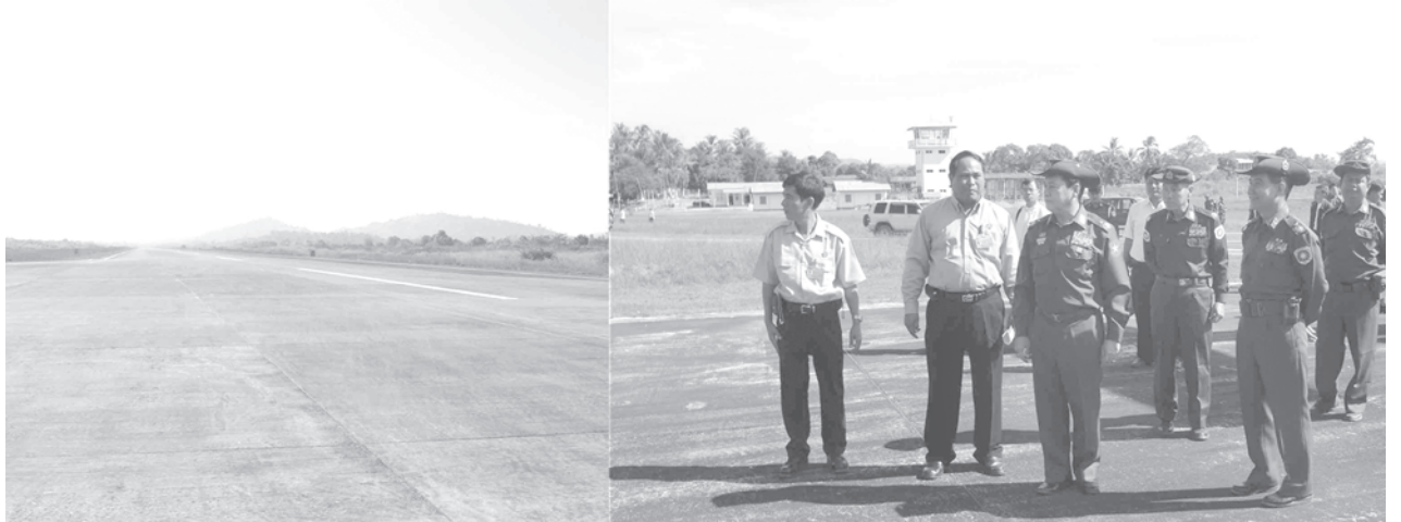
Commander Maj-Gen Thaung Aye and Minister Maj-Gen Thein Swe inspect runway of An Airport.—MNA
