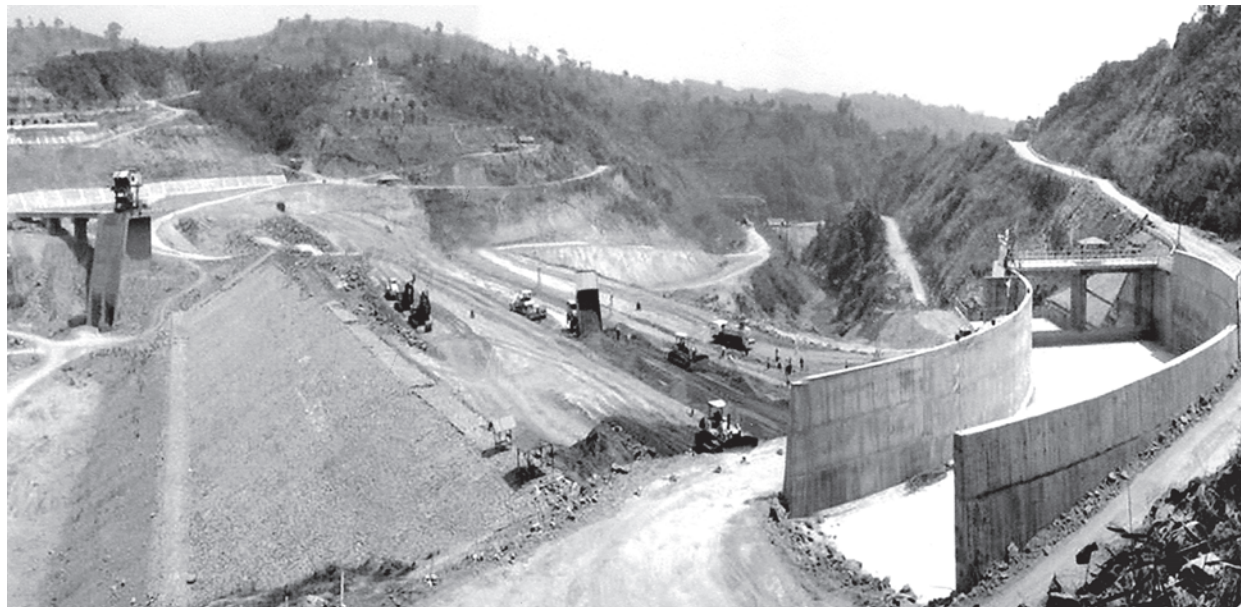
Main canal and spillway of Kunchaung Hydropower Project.
