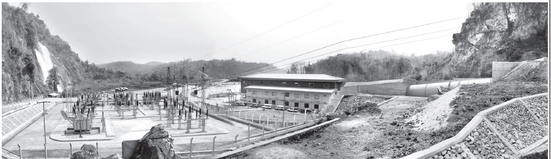
Photo shows progress in Kengtawng Hydropower Plant.
