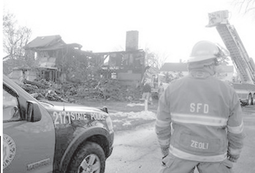
A firefighter stands in front of the remains of a house fire on 17 Fair St in Northampton, Mass, on 27 Dec, 2009. A father and son died in the house fire early on Sunday morning as firefighters struggled to put out more than a half dozen blazes, authorities said.
