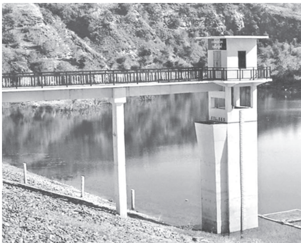
Control tower of Bawditahaung Dam.
