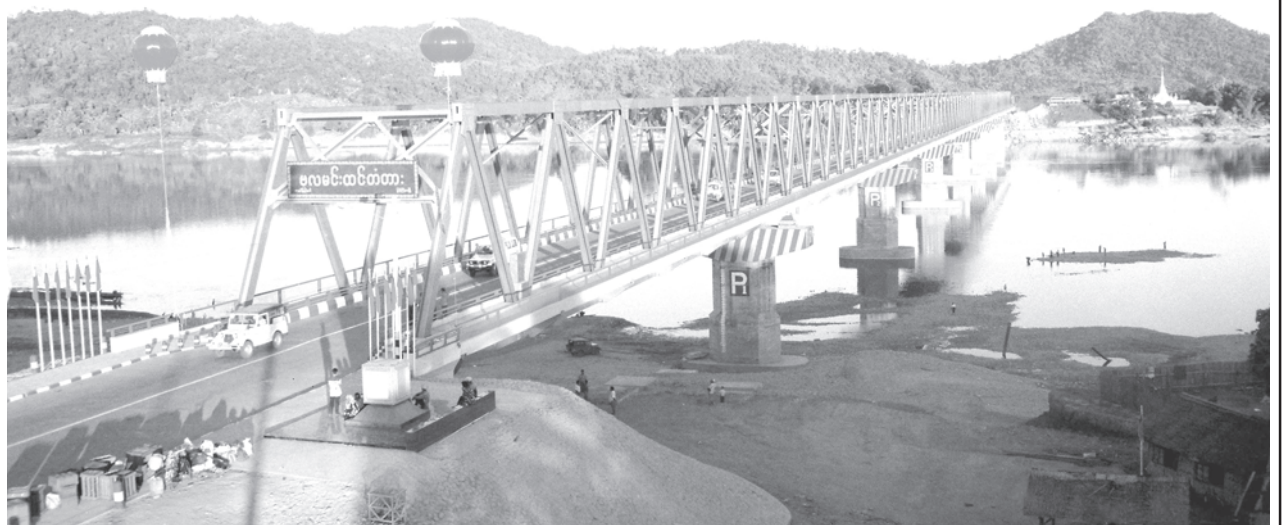
Photo shows Bala Min Htin Bridge.
