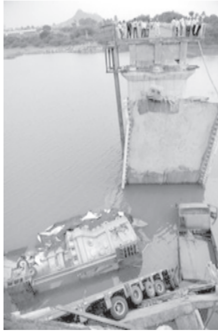
Officials from the Ahmedabad Fire and Emergency Services stand on the edge of a collapsed bridge in Talaja town, some 270 kms from Ahmedabad, in August 2009. At least 17 people were killed and 30 others were feared trapped or drowned after a bridge collapsed in western India, officials said on Friday.—INTERNET
