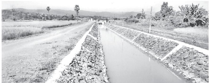
Main right canal of Ma Mya Dam.
