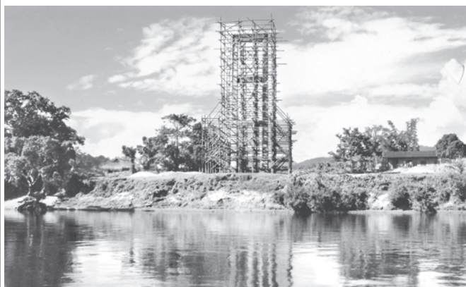
Kaunghmulon Bridge under construction over Malikha River near Kaunghmulon Village.
