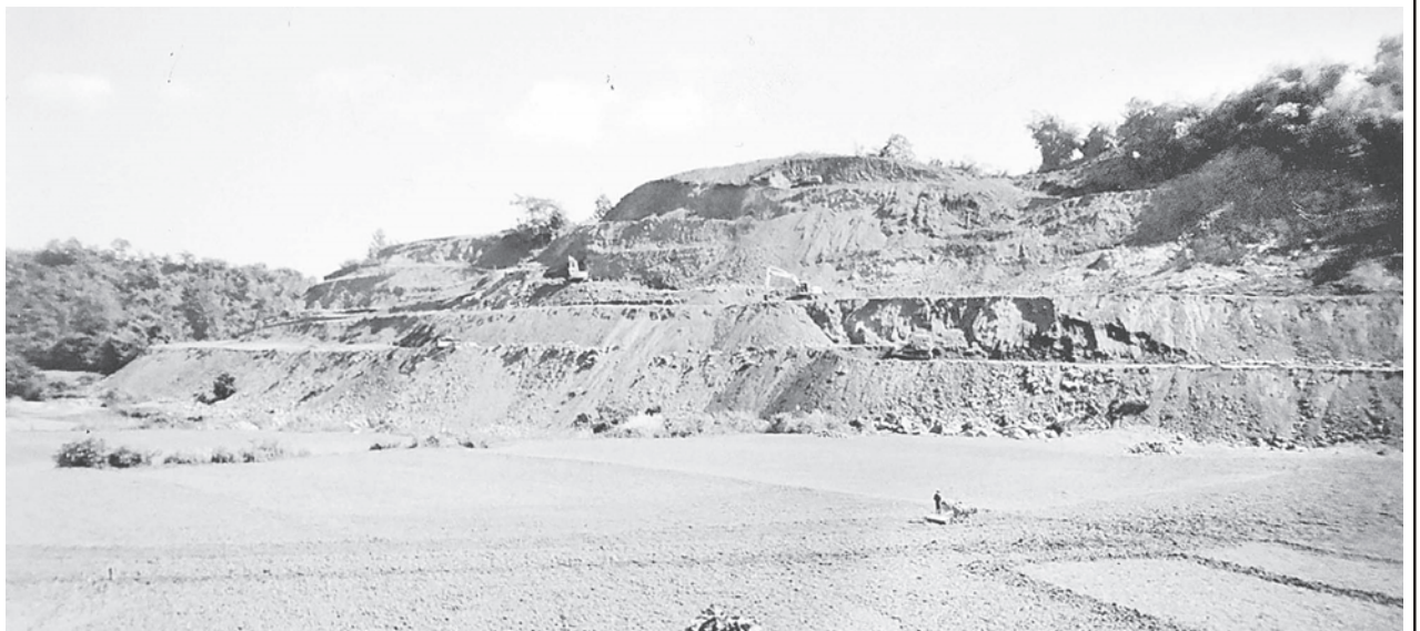
The construction site of the left main canal.
