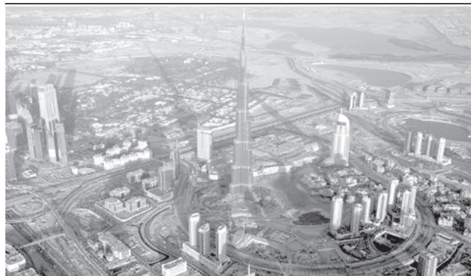
An aerial view of the Burj Dubai, the world's tallest tower, in Dubai on 21 Dec, 2009. State-owned Dubai World did not ask creditors for a standstill on $22 billion of debt at a meeting on Monday, adding to uncertainty for investors who have been in the dark for weeks and hurting local bank shares.—XINHUA
