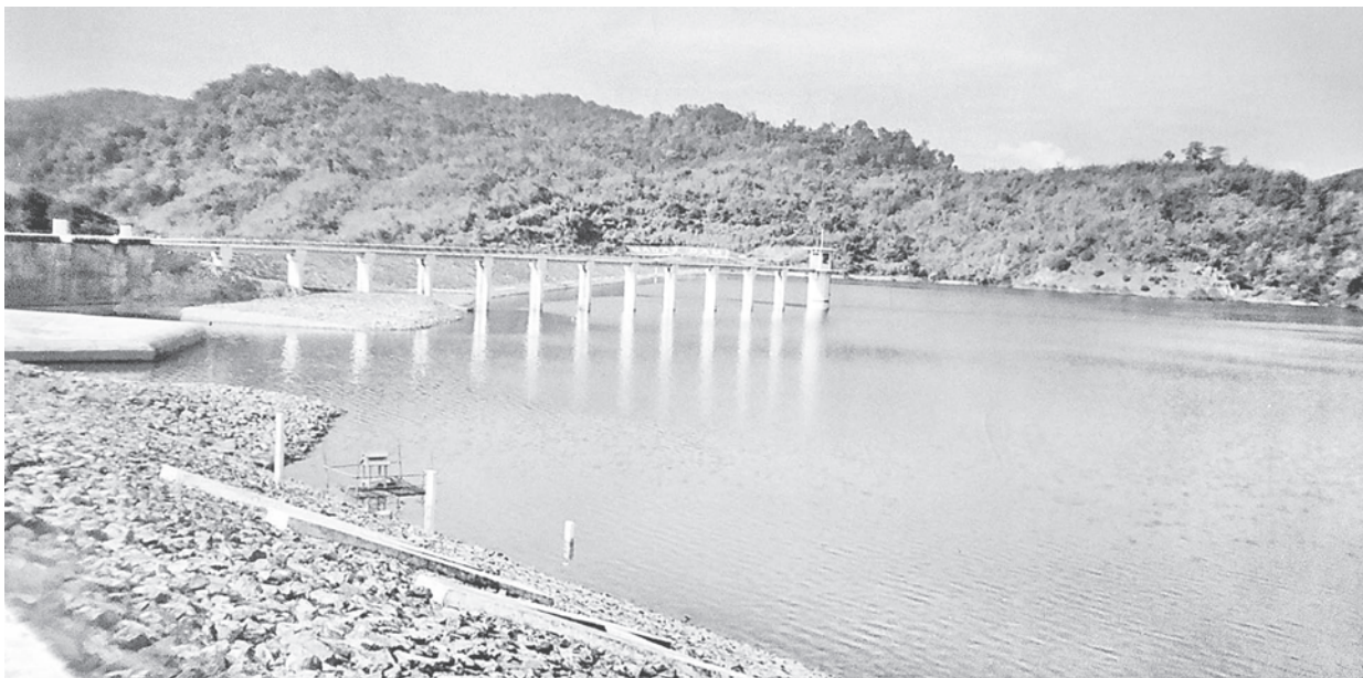
Maday Dam with its control tower in Kanma Township, Magway Division.
