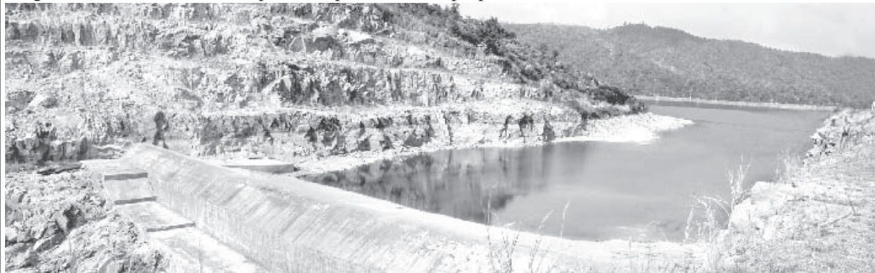
Photo shows the spillway of Paunglaung multi-purpose dam.
