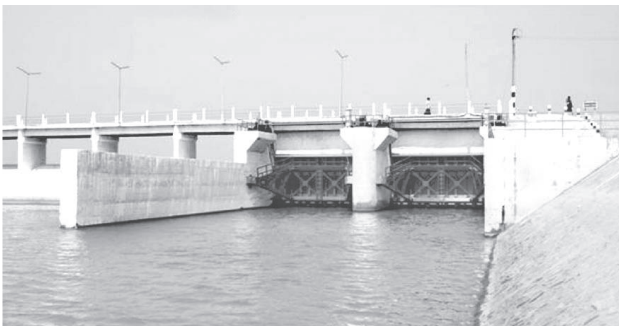
Diversion weir of Paunglaung multi-purpose dam.
