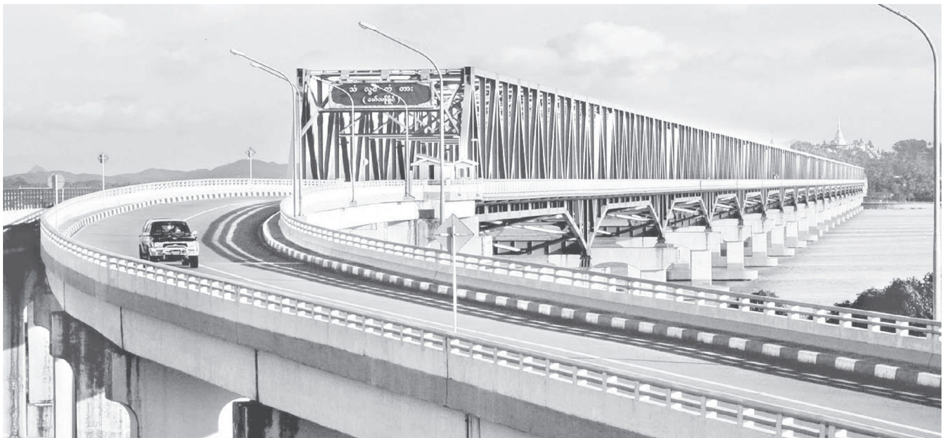
Photo shows Thanlwin Bridge (Mawlamyine).
