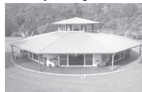
An octagonal, three-bedroom, family home built on a rotating platform near Wingham, about 250km (155 miles) north east of Sydney, is shown in this undated handout picture. The house, which cost about A$700,000 ($641,000) to build, can complete a full rotation in about 30 minutes according to its owners.
