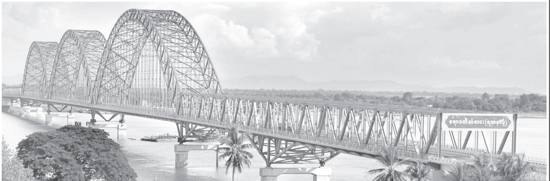
Photo shows magnificent Ayeyawady Bridge (Yadanapon).
