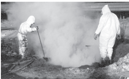
In this on 7 Dec, 2009 picture provided by the Alaska Department of Environmental Conservation, crews use steamer equipment to melt contaminated material for collection with a vacuum rig.—INTERNET
