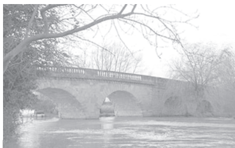
The 242-year-old Swinford Toll Bridge, Oxfordshire, seen here, whose owner can earn tax-free income was sold at auction.
