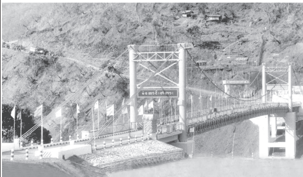
Photo shows Manhsaung Bridge in Tiddim Township, Chin State.
