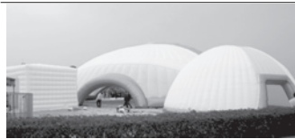
Photo taken on 2 Dec, 2009 shows a triplet of super air inflatable tabernacles, standing at a height of 10 metres, 5 metres, and 4.6 metres, respectively, on the cultural square of Wuyuan County, east China's Jiangxi Province. The PVC-quality air tents, a product developed by a local producer, are equipped with air-conditioning, electrical circuits, and other facilities, and capable of fire-prevention and earmarked for occasions on exposition, celebration, etc. The three tents has been reserved for an order from Great Britain.
