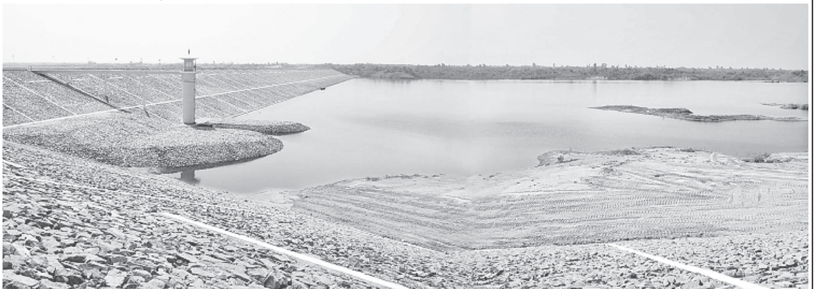
Wakadoke Supporting Dam situated near Taungset-in Village, Bago Township of Bago Division.
