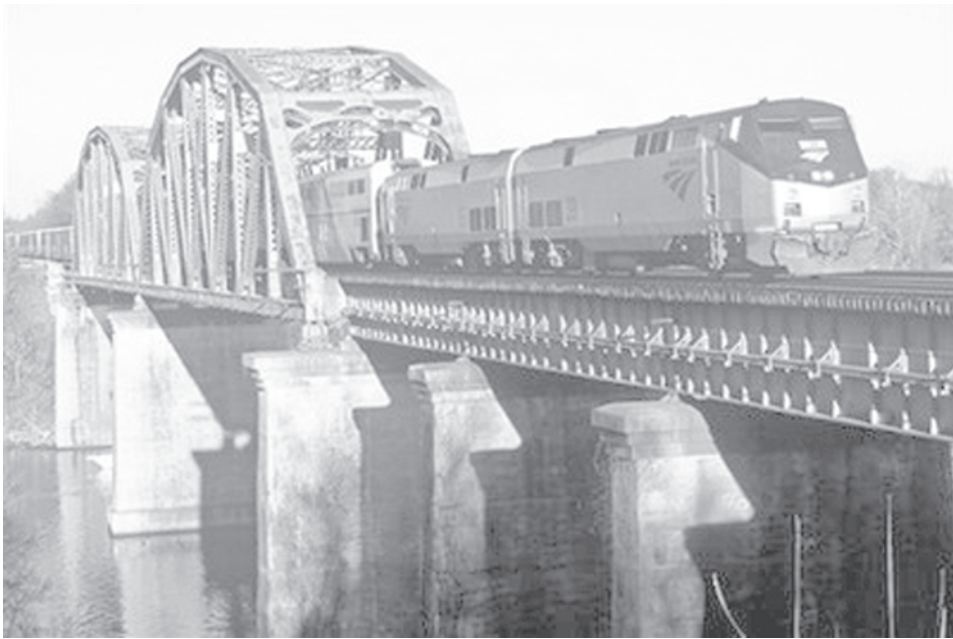
This undated photograph provided by Amtrak shows an Amtrak Auto Train crossing a bridge in Woodbridge, Va.—INTERNET
