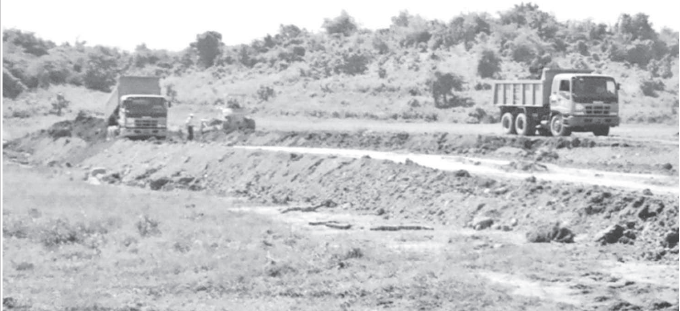
Water supplying canal being constructed with the use of heavy machinery.
