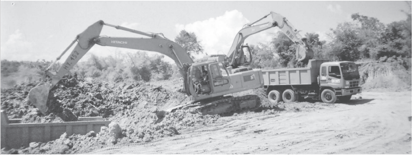
Groundwork is being carried out with the use of heavy machinery.
