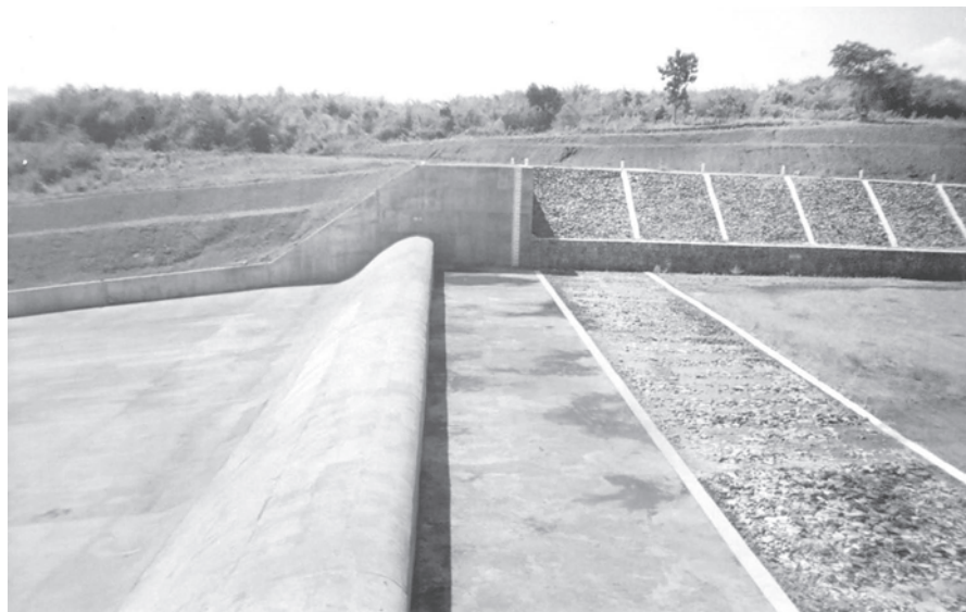
Completed spillway of Kanyin Dam.
