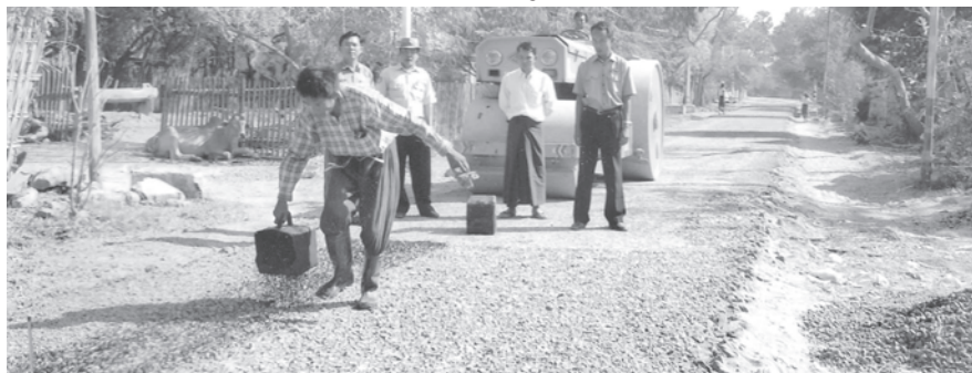
Upgrading of Thitsar Street into tarred one in progress.
