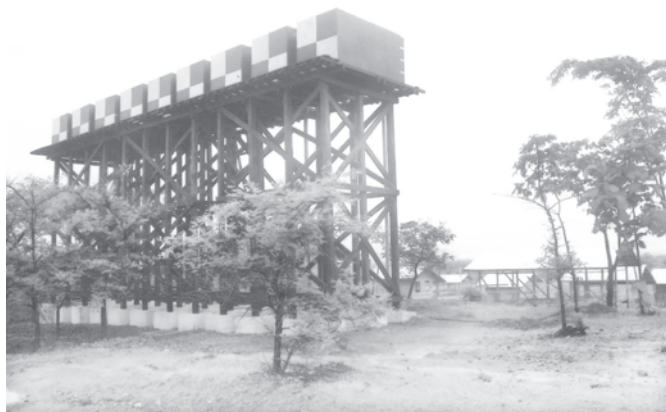
A row of 7200-gallon overhead tanks.
