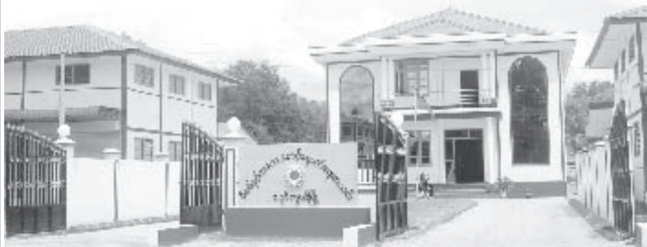
Newly-built Pyawbwe Township Maternal and Child Welfare Association Office.
