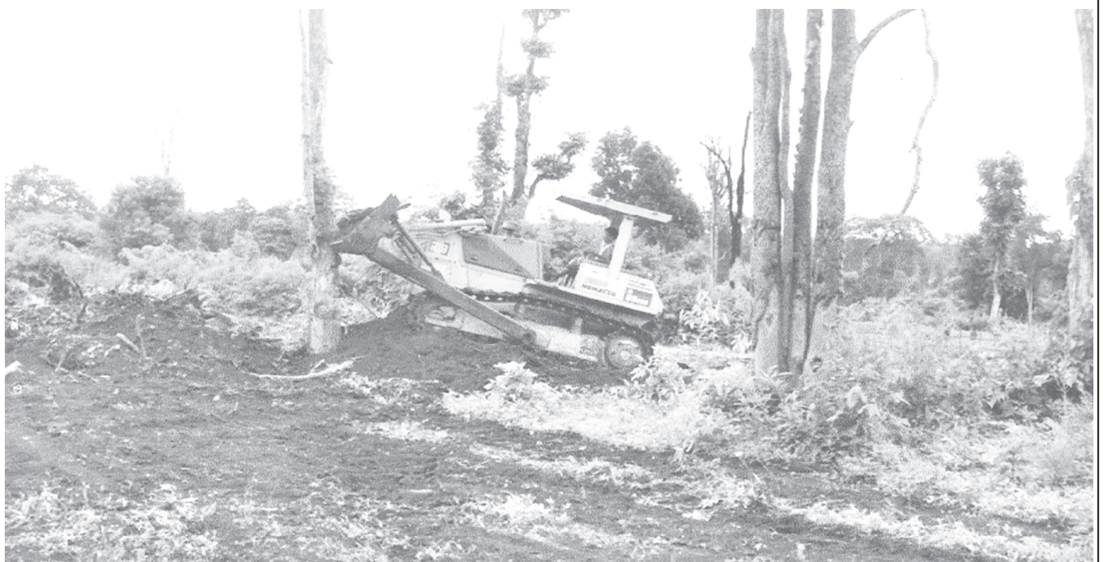
Clearing the site with heavy machinery in Nantpapaung Dam construction project.
