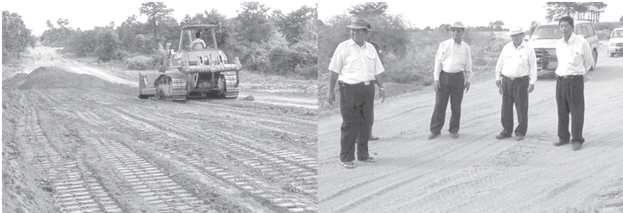
Deputy Minister U Tint Swe inspects earthworks on Patheinywa road.—CONSTRUCTION
