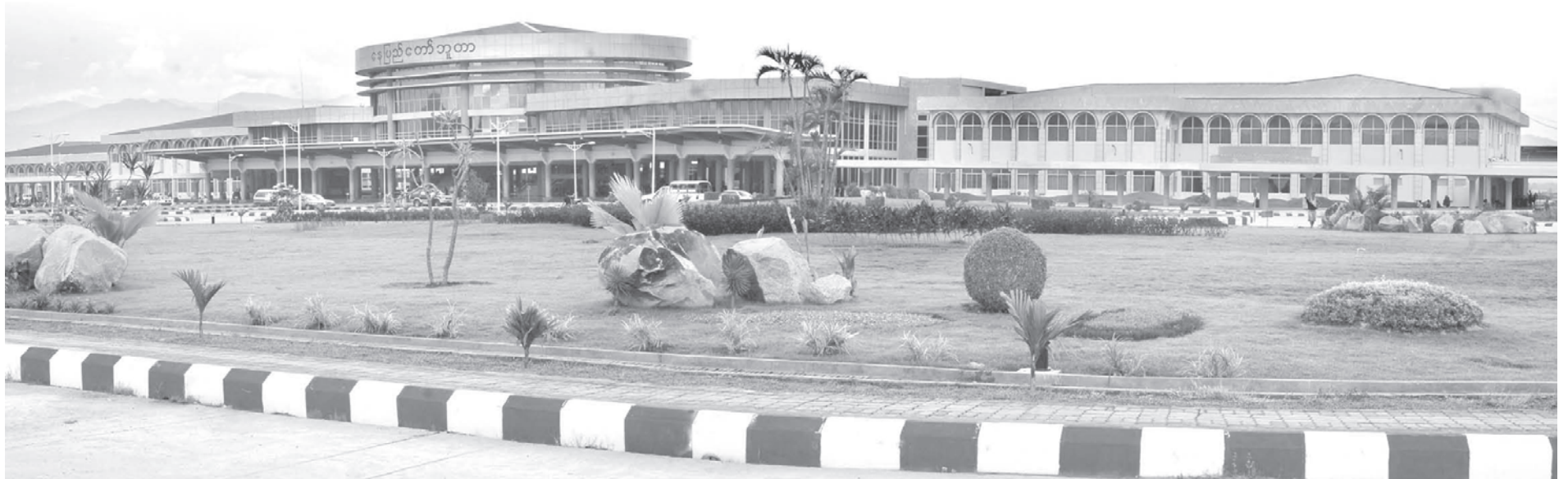
Photo shows newly constructed Nay Pyi Taw railway station.
