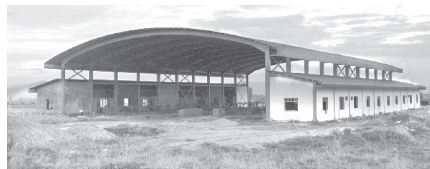
Locomotive shed under construction.
