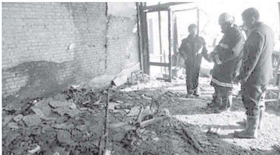
Firefighters work at the restaurant that on fire in Qingyun County of east China's Shandong Province, on 19 Nov, 2009. Six people were killed and three injured early Thursday after a restaurant went on fire in Qingyun County, local authorities said.—XINHUA
