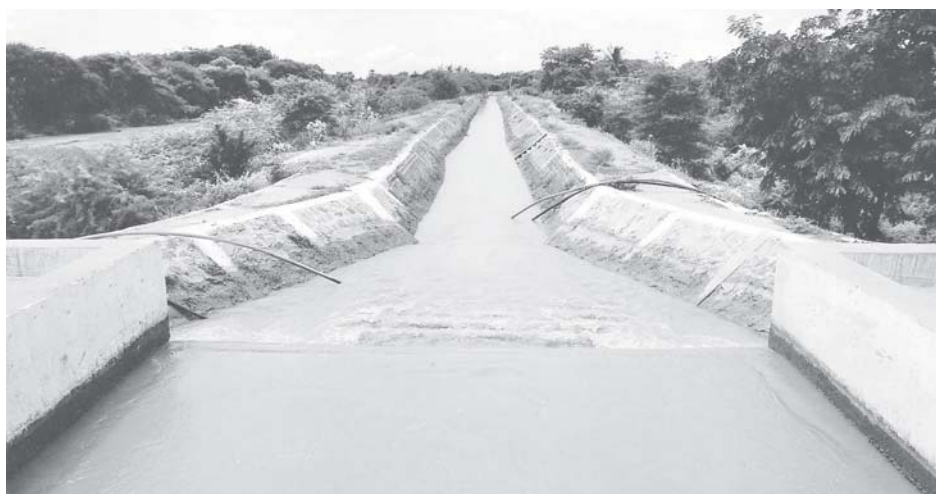
Photo shows six feet wide, six feet deep and 26,950 feet long main canal of water pumping station.
