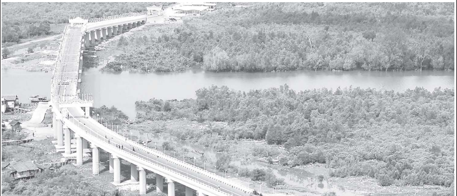
Photo shows Minkyaung Bridge on Maei-Kyaukpyu Road Section.
