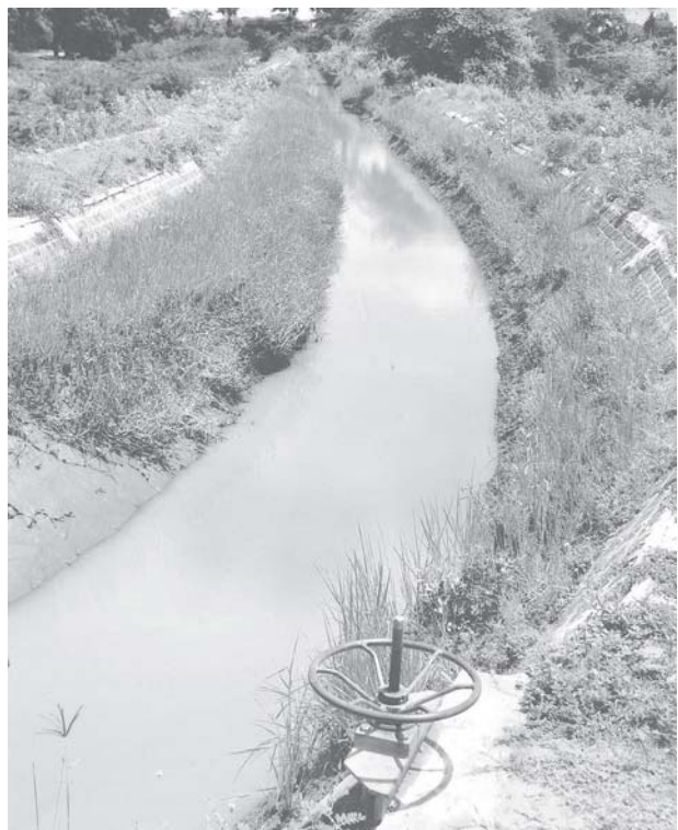
Irrigation water flows in five feet wide, four feet deep and 68,900 feet long tributary canal of water pumping station.
